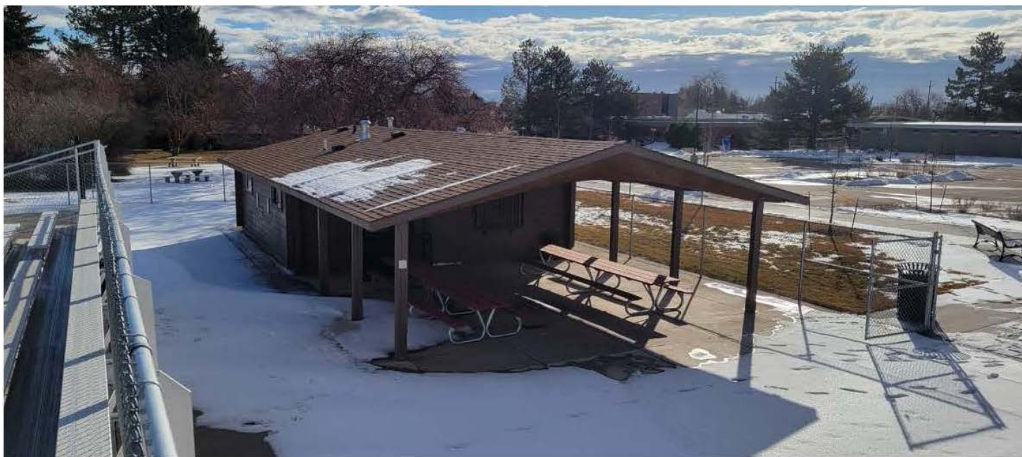
BUTCH BUTLER 3 - Existing concession / restroom (original building purchased via Sears Catalog).
