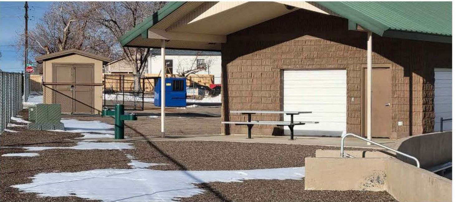
FORBES 4 - Existing concession / restroom (mid-ground) and storage shed (background).
