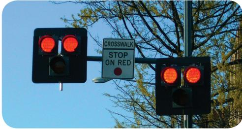
A **HAWK** (High-Intensity Activated crossWalk) signal is a signal-beacon designed to help pedestrians safely cross busy streets.
