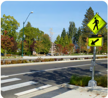
Installation of rectangular rapid flashing beacon pedestrian crossing signs
