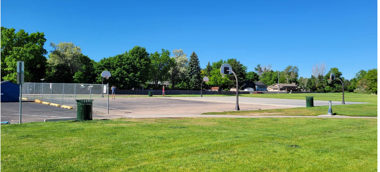
BITTERSWEET 3 - Existing basketball courts lacking shaded seating and perimeter fencing.
