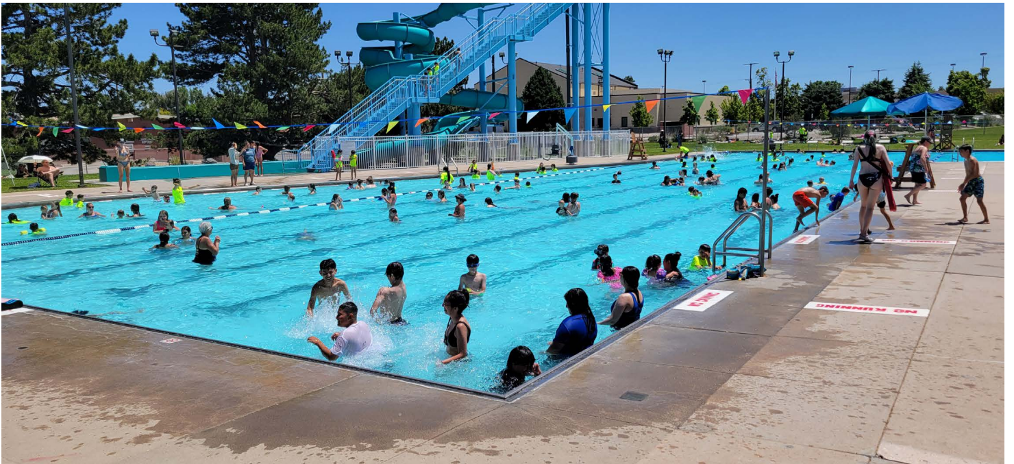
CENTENNIAL POOL 1 - Existing pool in need of repairs and deepening for competitions.
