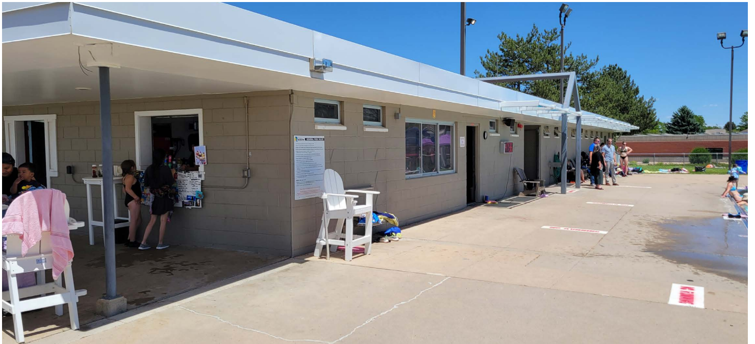
CENTENNIAL POOL 2 - Existing concession / restrooms.
