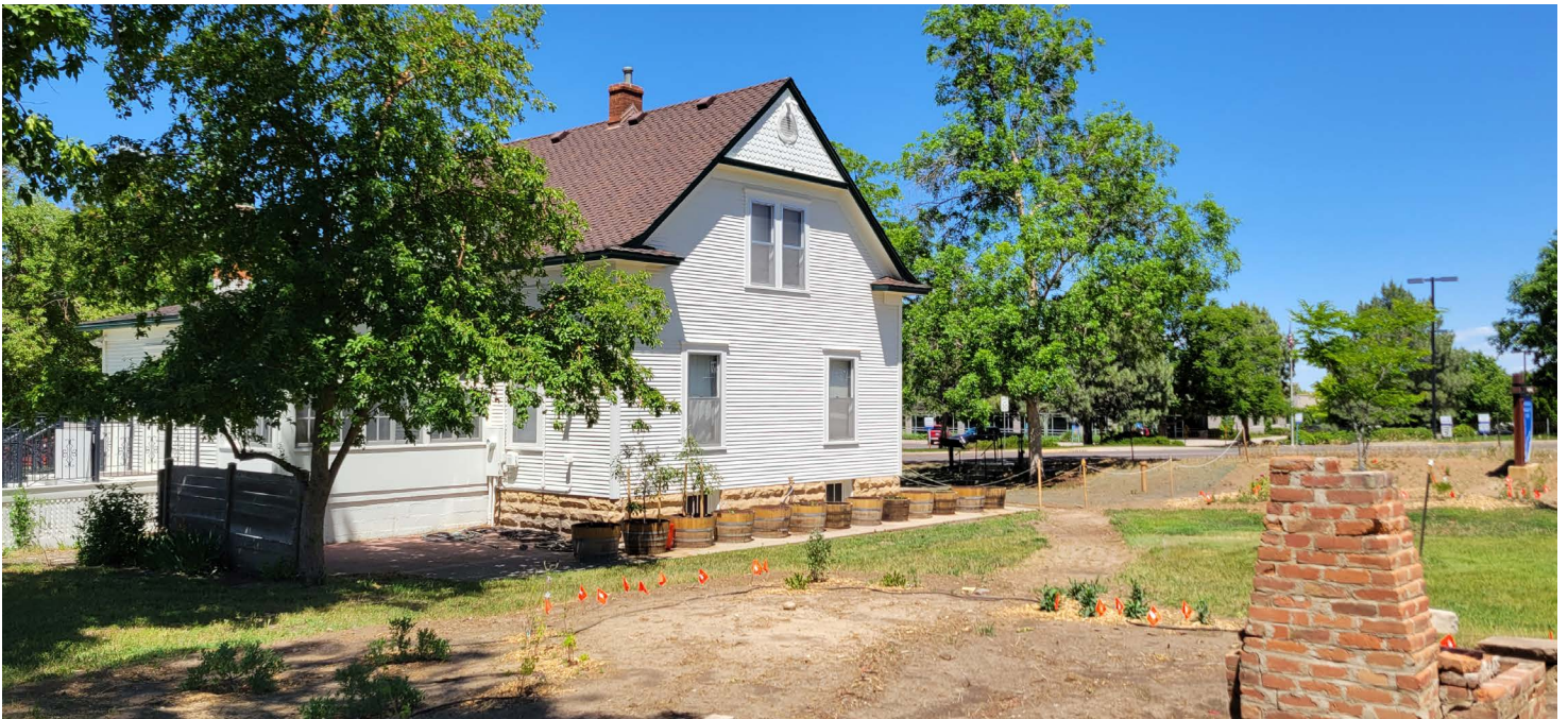
WHITE PLUMB 1 - Existing farmhouse.
