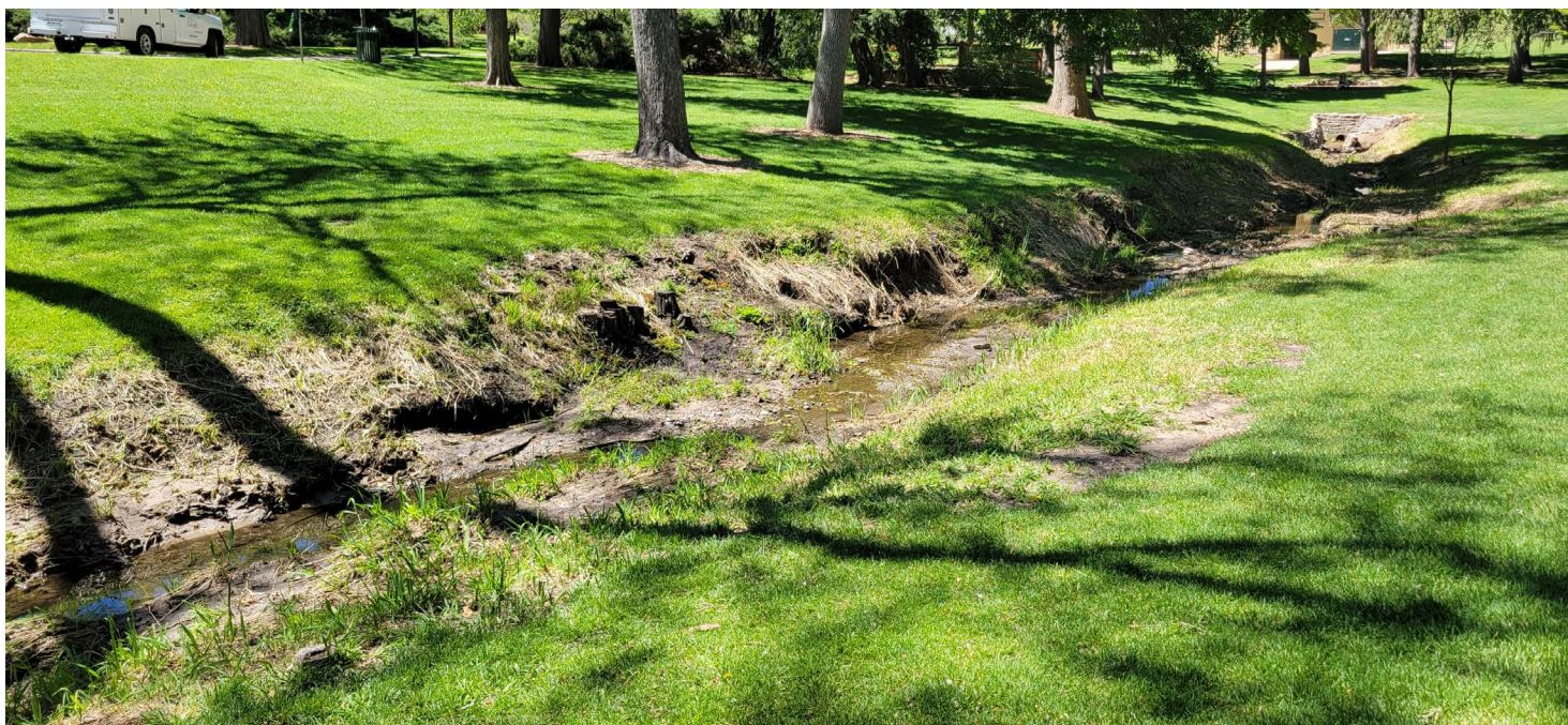
GLENMERE 5 - Erosion at existing channel draining into pond.
