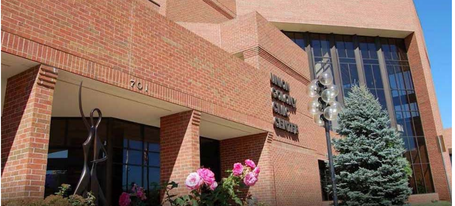
UCCC 1 - Main entry signage in need of improvements to differentiate building from adjoining Recreation Center.
